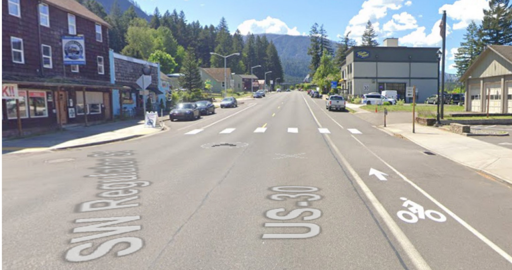
Figure 7.10 Wa Na Pa St. and Regulator St., Cascade Locks Stage 1 (Base)
