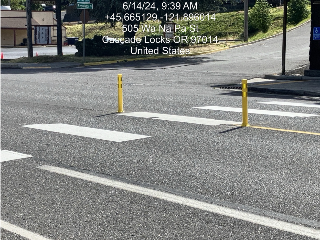
Figure 7.11 Wa Na Pa St. and Regulator St., Cascade Locks Stage 2 (Post on CL)
