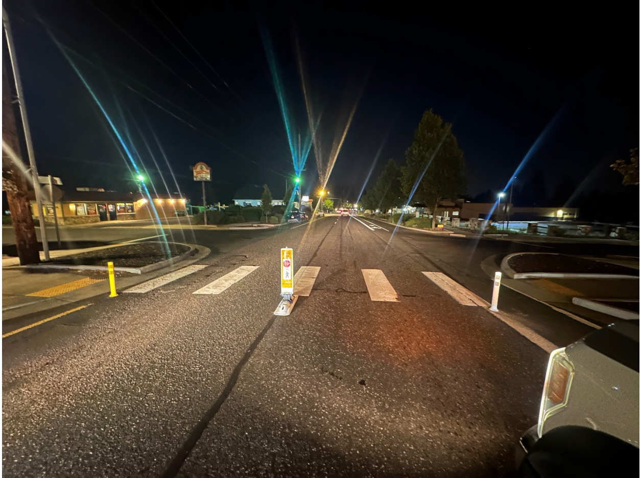
Figure 7.28 Proctor Blvd. and Beers Ave, Sandy Stage 4 (R1-6a + Post)
