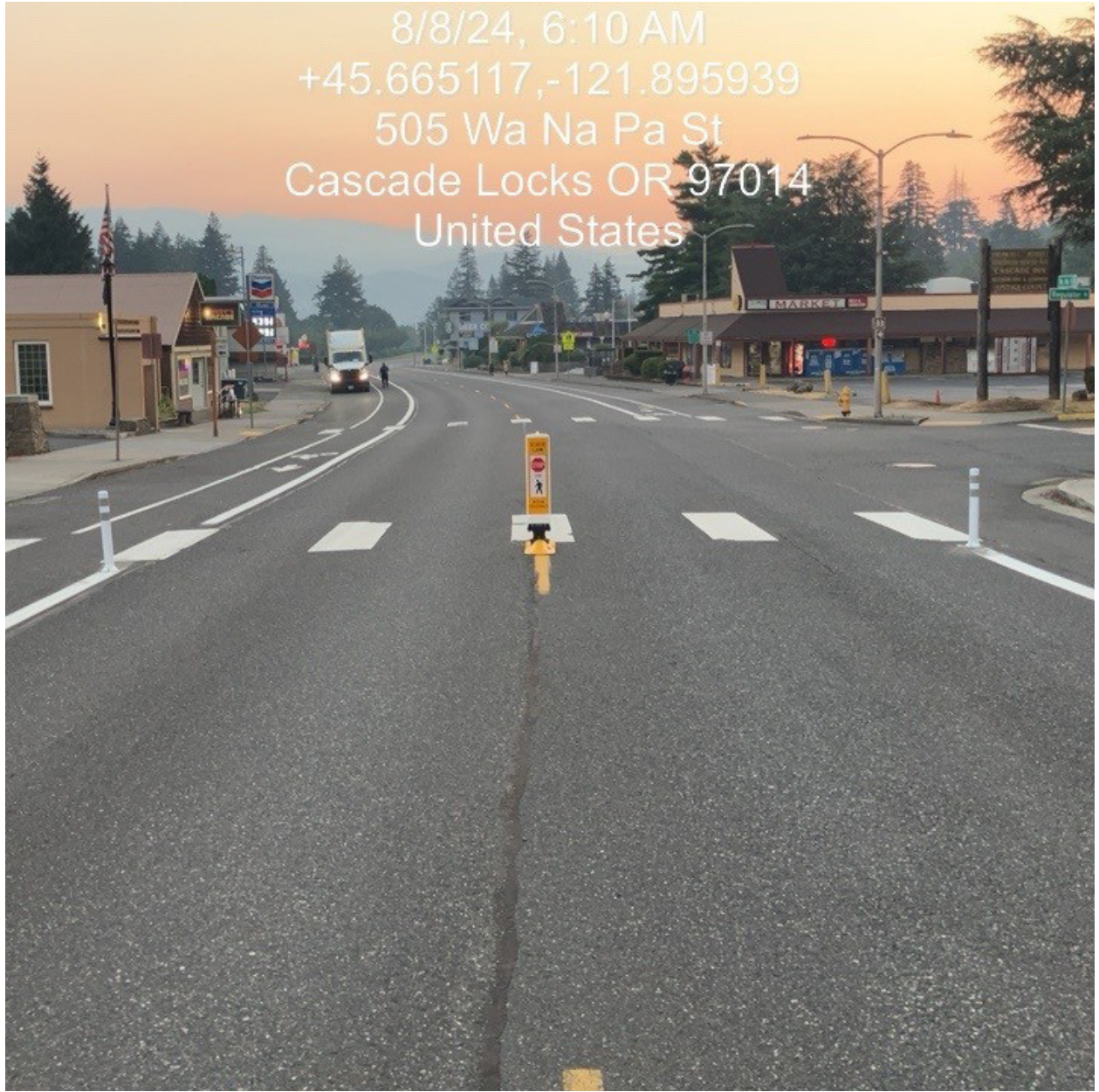
Figure 7.13 Wa Na Pa St. and Regulator St., Cascade Locks Stage 4 (R1-6a + Post)
