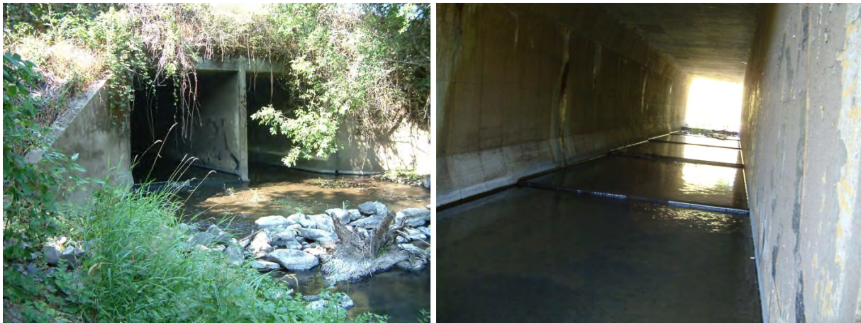
Figure 4.6: Site 04 – Oak Creek downstream and structure
