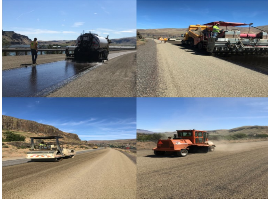
Figure 9.3. Chip seal construction equipment
