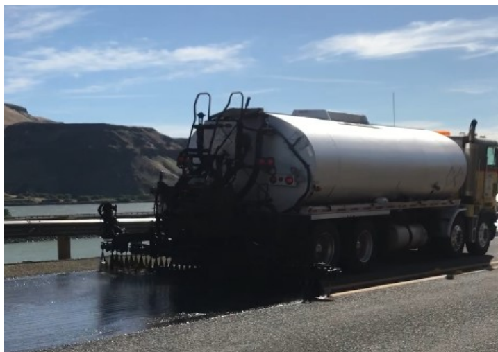
Figure 9.5. Asphalt emulsion spraying for triple coverage
