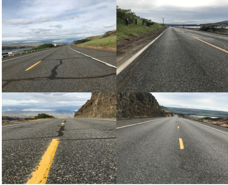
Figure 9.2. Road condition before chip sealing on Oregon 206
