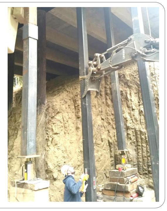
Step 10: Preload with 20 ton hydraulic jack
