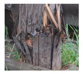
• Installing steel sleeves to hold the pile together can buy some time.
