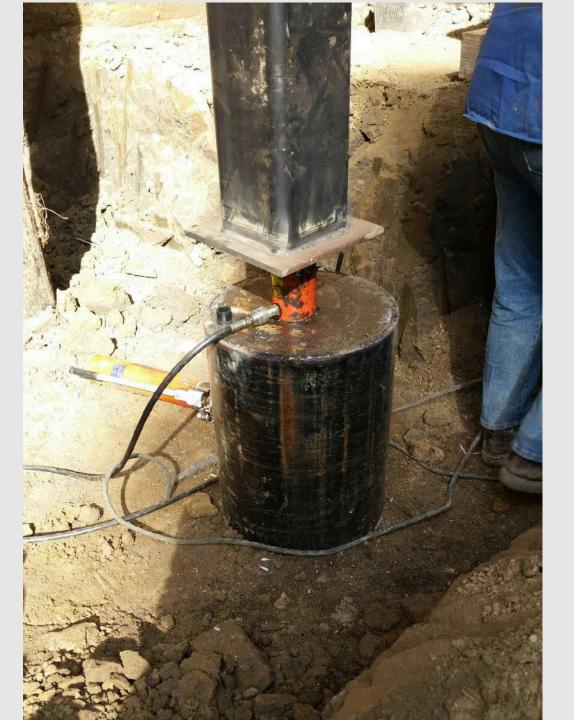
Step 11: Cut shims to fit and weld in place.
