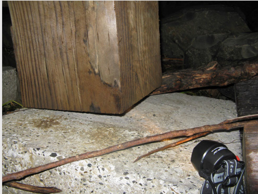
Debris between column & footing
