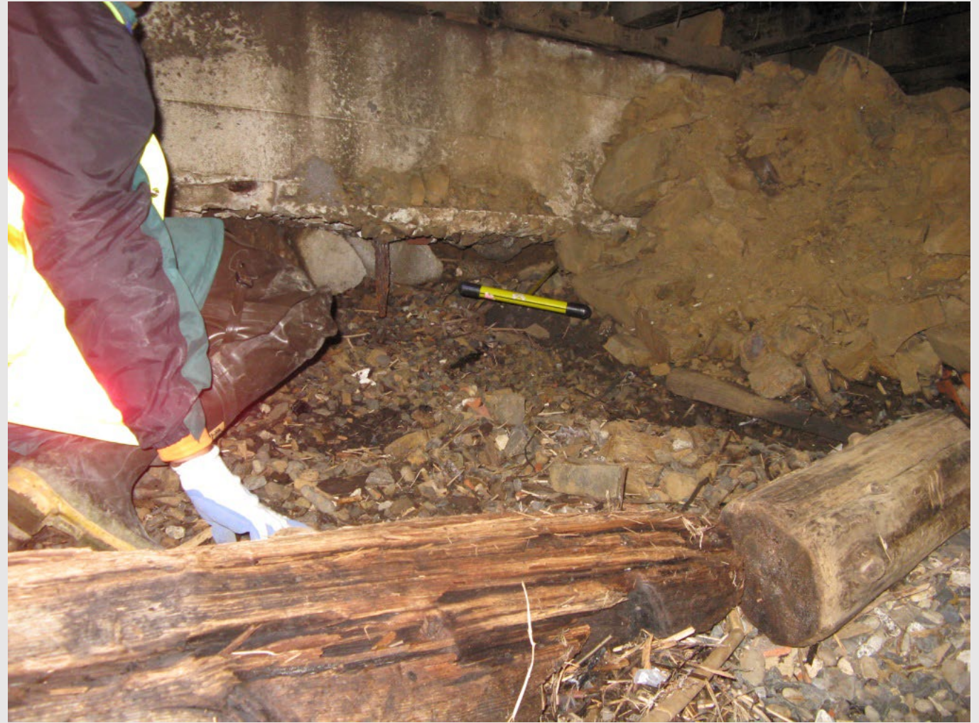
Debris between column & footing
