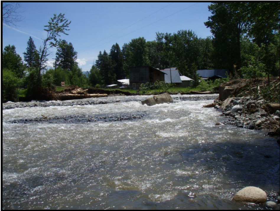
Gulick Road bridge failure.
