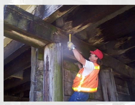
sounding the wood surface by striking it with a <u>3lb</u> <u>hammer</u> or other object and based on the tonal quality of the sounds, a trained inspector can interpret dull or hollow sounds that may indicate the presence of large interior voids or decay.
