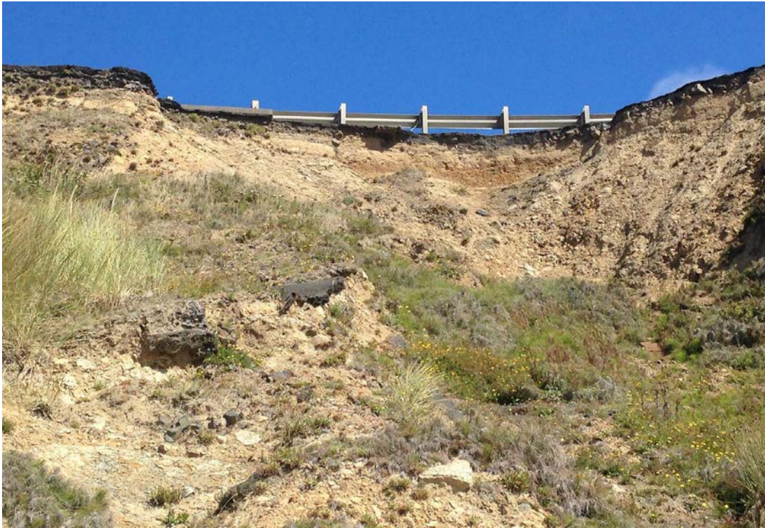
Wave action from storms has eroded away areas of roadway asphalt and is close to compromising the guardrail along US 101, southbound lane. Credit: ODOT.
