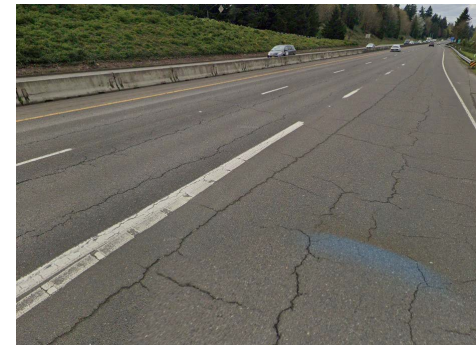
Cracking and rutting on the OR 224 pavement
