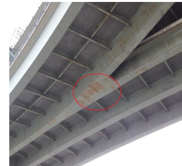
Rust on the underside of the Fremont Bridge ramp.
