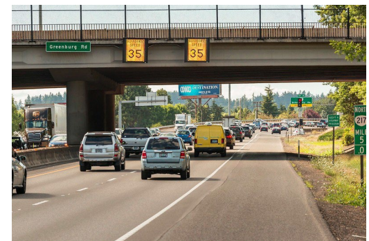
Example of variable speed signs on OR 217
