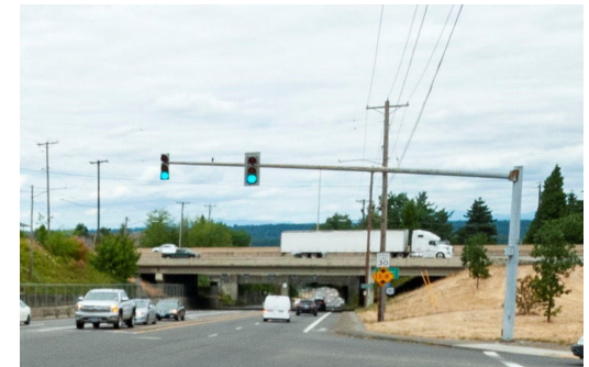
An example of a small, non-standard signal head
