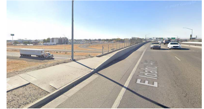
Barrier separating sidewalk from U.S. 30 over I-84
