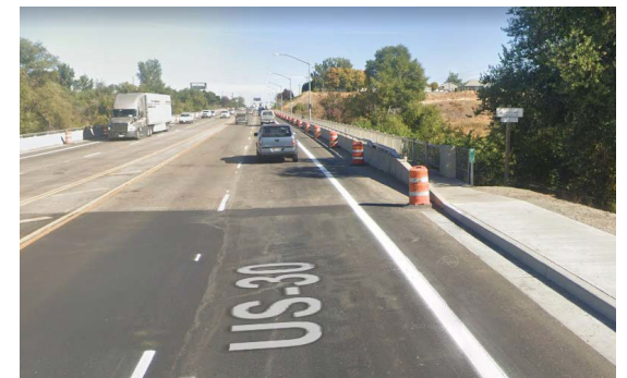
Barrier separating sidewalk from U.S. 30 over I-84
