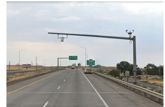
Weigh-in-motion on I-82, milepost .89, south of the Oregon/Washington state line. The device captures axle and gross vehicle weights as vehicles drive through site.
