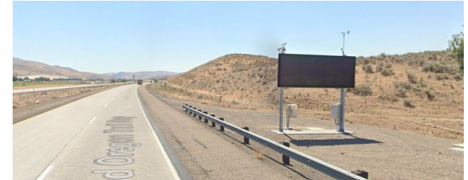
Variable message sign (VMS) along I-84. Electronic roadside signs inform drivers in advance of incidents and other useful road conditions or travel information.
