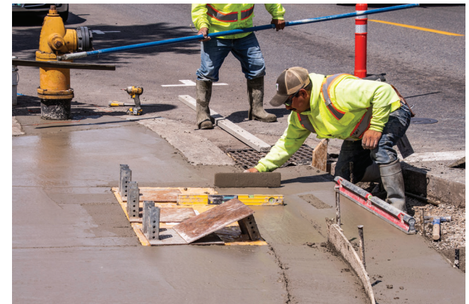
Top photo shows crews pouring concrete, bottom photo shows crews smoothing concrete for ADA compliant curb ramps.
