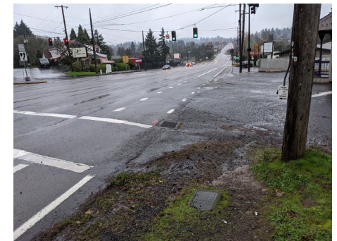
Existing conditions: OR 99W at SW 24th Ave
