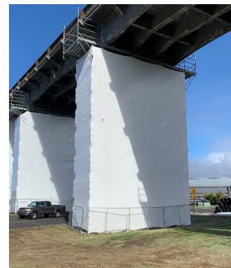
Scaffolding and enclosure examples.
