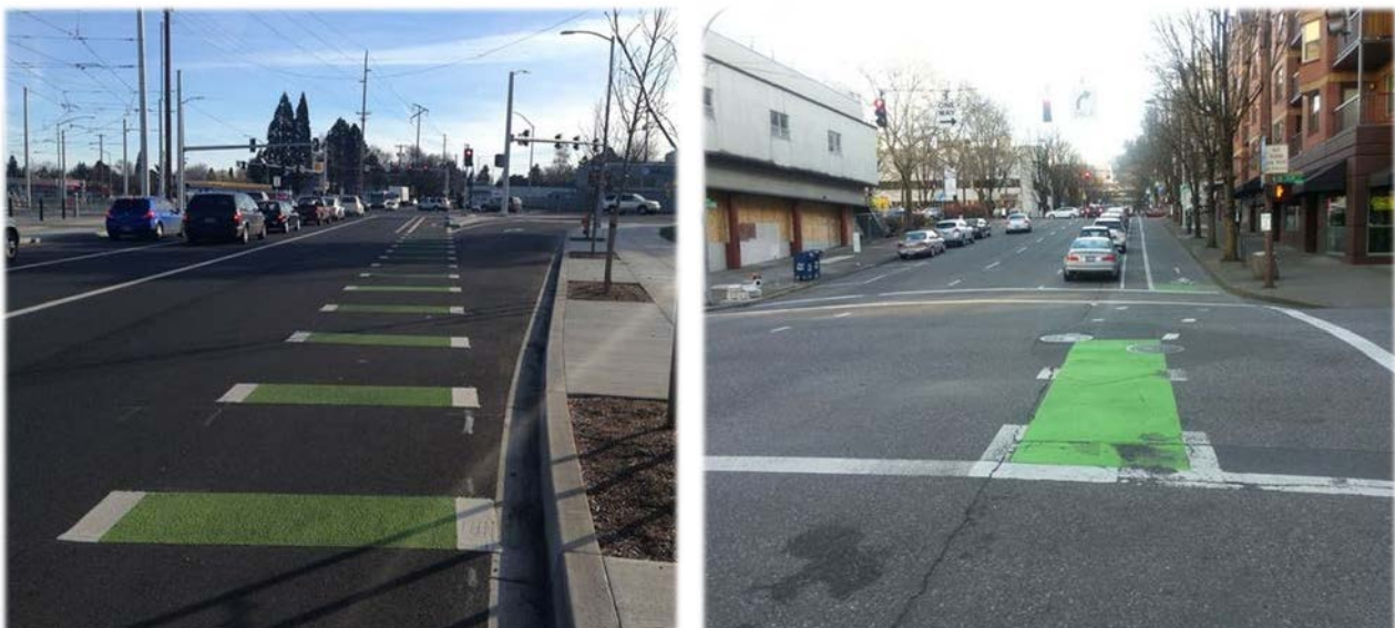
Exhibit 23. Non-corridor example green paint through a turn lane and through an intersection (Portland, OR)
