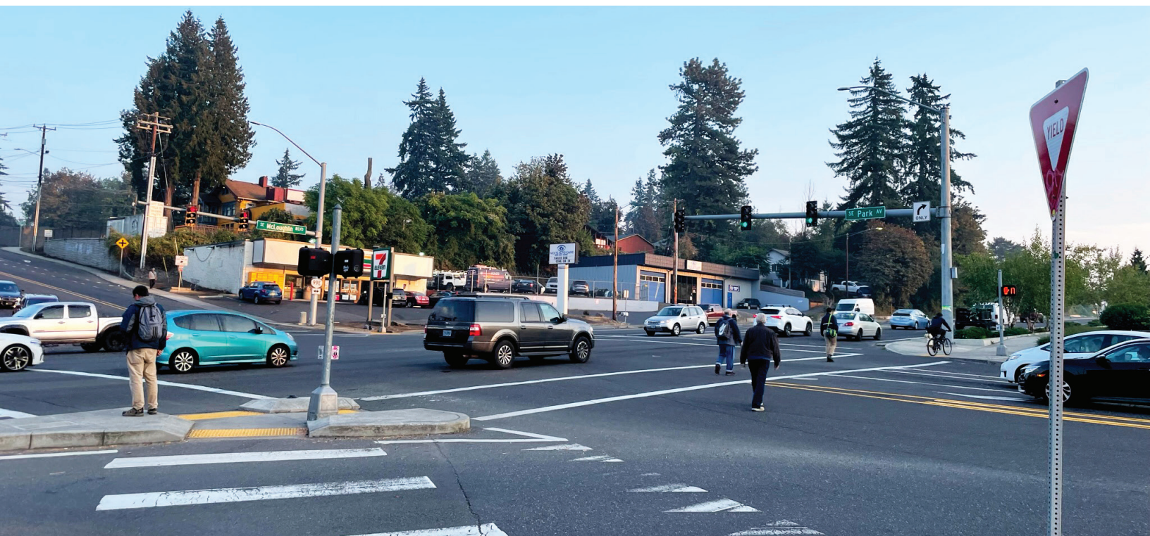
2023 – Crosswalks see heavy use at the intersection of McLoughlin Boulevard and Park Avenue. Adjacent to the Park Avenue MAX Station.
