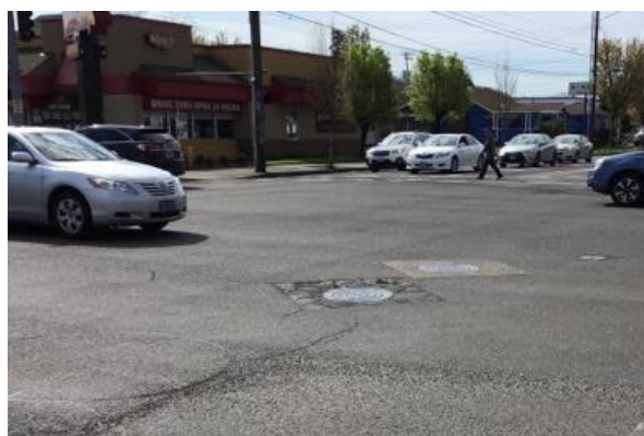
Concrete around utility cover is broken (poor)
