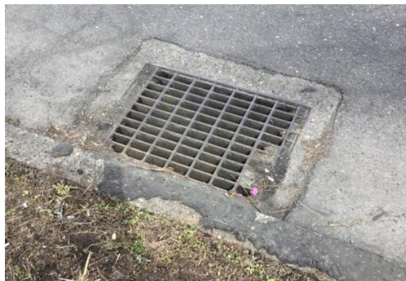
Pavement around drainage inlet is uneven (fair)
