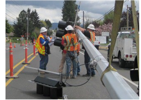
ODOT crews installing a new traffic signal
