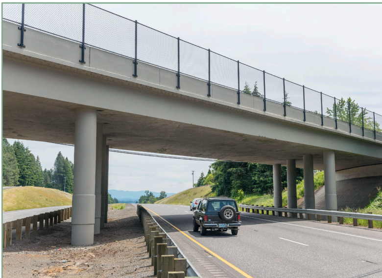
An example of protective screening similar to what ODOT will install on both sides of the N Ainsworth Street bridge over I-5 in Portland beginning in July.
