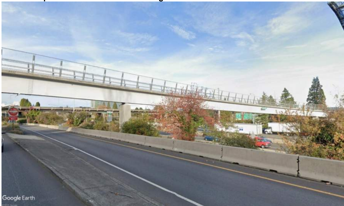
Figure 3. Example of a Girder Pedestrian Bridge
