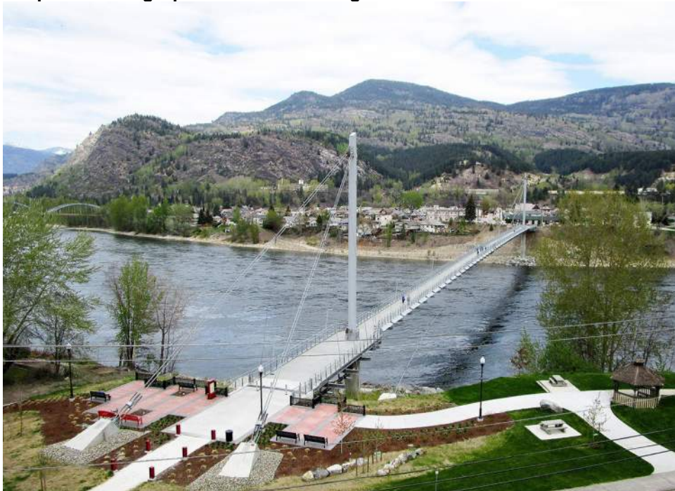
Figure 2. Example of a Long-Span Pedestrian Bridge
