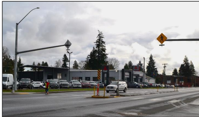
Potential Crossing Treatment - Overhead RRFB
