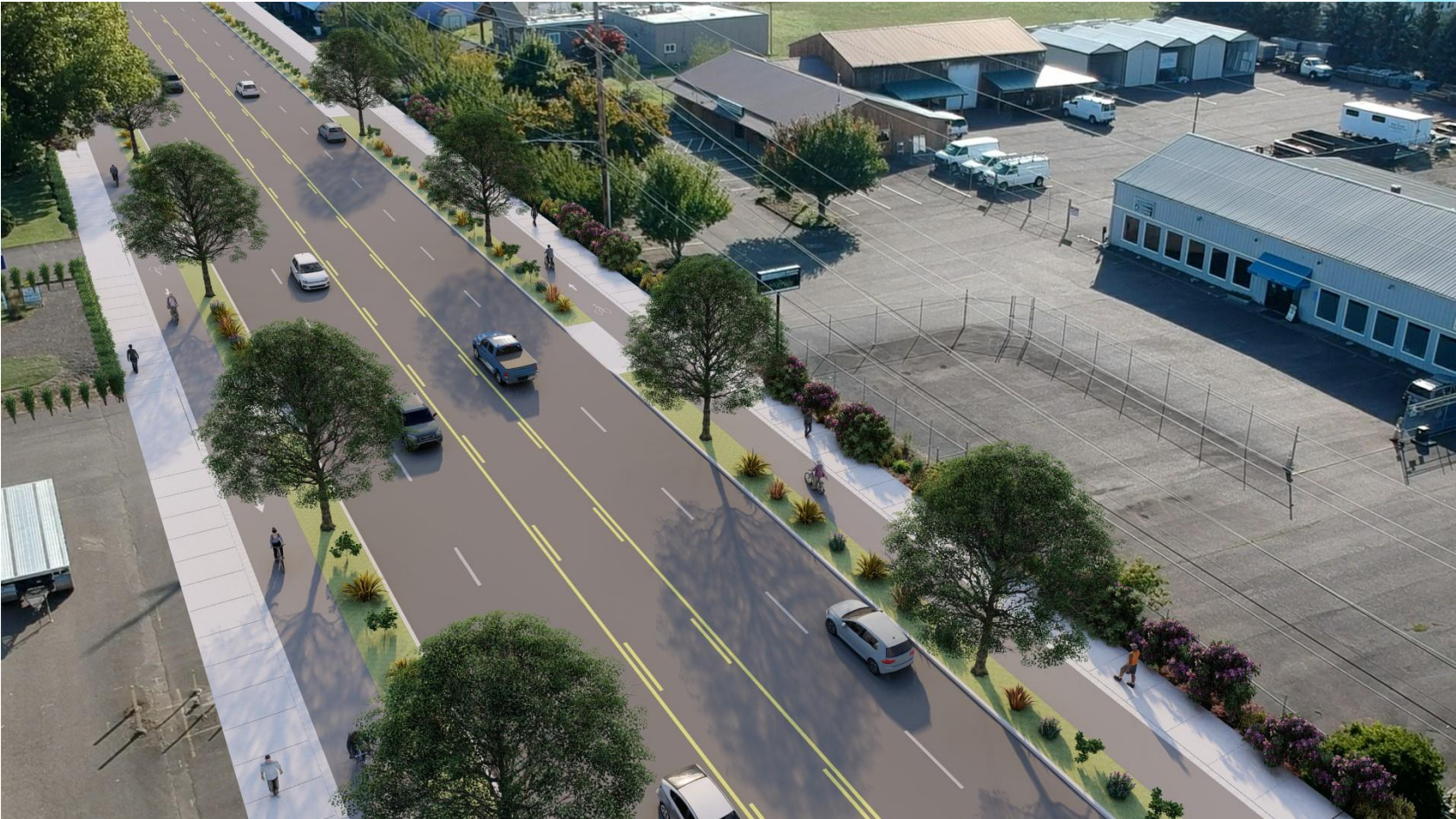
Transition from 5 lanes to 3 lanes to occur between Prairie Ave and Goodnight Ave.
