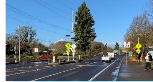
Potential Crossing Treatment - RRFB
