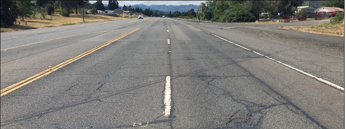
**Pavement:** The four-mile area of Oregon 42 between Lookingglass Creek and Grant Smith Road was last paved in 2006. The pavement shows extensive surface wear and cracking. Turns lanes are heavily rutted.
