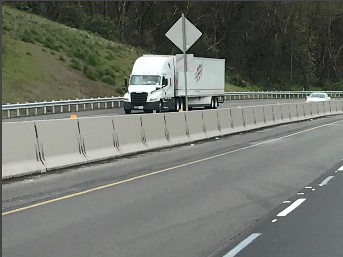
To help reduce the number of crashes involving turning movements and lane departures, ODOT will place raised concrete barrier (similar to that seen in the photo) along some areas of the Oregon 42 median.
