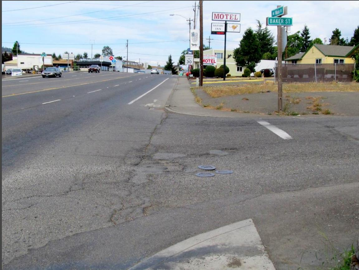
In addition to replacing ADA curb ramps, ODOT will also pave crosswalks and side street approaches, like this one at Baker Street, that are damaged or heavily cracked.
