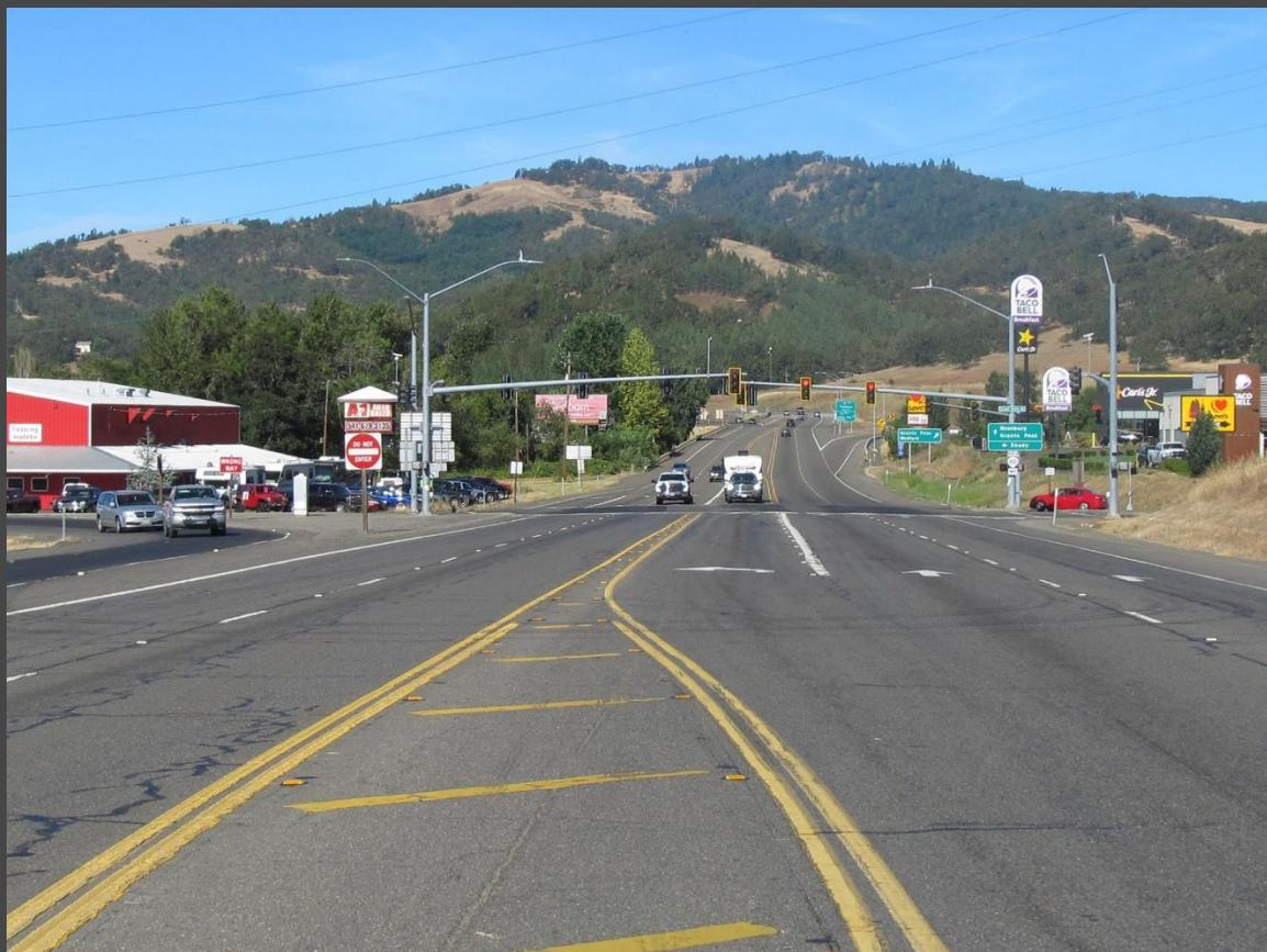
At the Grant Smith Road intersection, ODOT will install raised traffic separators and concrete islands along the center median, adjust the roadway to better accommodate U-turns, and upgrade sidewalk curb ramps.
