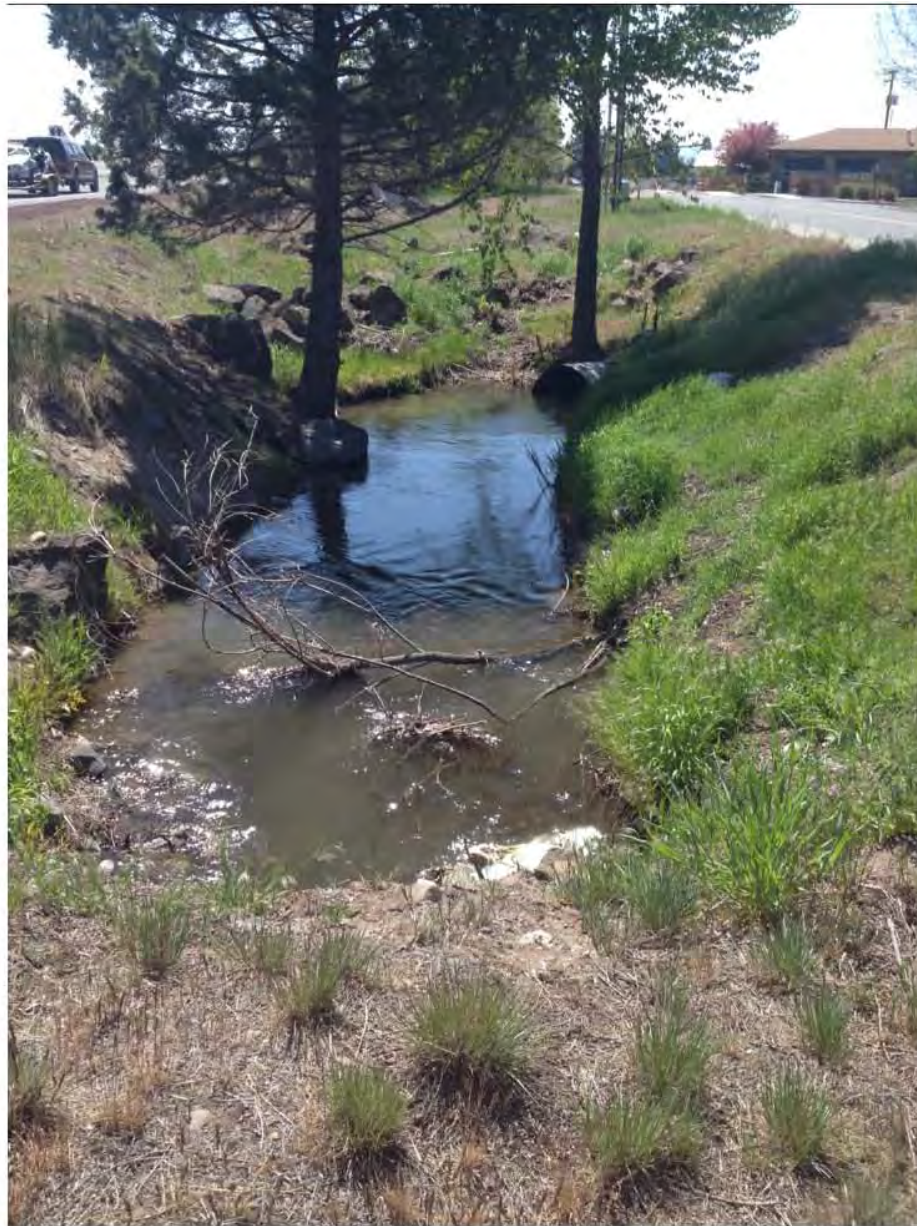
Figure 3: Swalley Rogers Lateral at Xanthippe Lane (to be piped) looking east. No historic features were found that reflected early construction, or detailing – this lateral has been subject to more recent corrugated metal piping (CMP) under adjacent roads (May 15, 2014).
