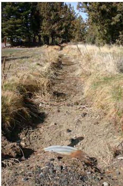
View: Corrugated metal pipes were commonly used as culverts for the Rogers and Riley canals, as was observed at the crossing of the Rogers Canal at Cooley Road. The view is towards the north.
