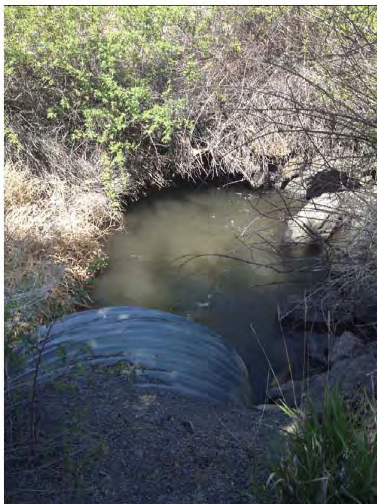
Figure 7: Swalley Rogers Lateral: US97 – US20 Segment D (to be piped) view to the west. No historic features were found that reflect early canal construction, or detailing and the lateral has been subject to more recent corrugated metal piping (CMP) under the adjacent roads. (May 15, 2014)
