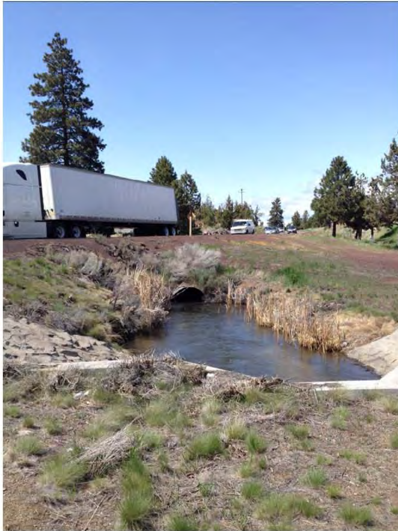
Figure 5: Swalley Rogers Lateral: US97 – US20 Segment B (to be piped) looking to the northwest. No historic features – the concrete retaining wall in foreground is of relatively recent origin – were found that reflected early construction, or detailing and the lateral has been subject to more recent corrugated metal piping (CMP) under the adjacent roads. (May 15, 2014)
