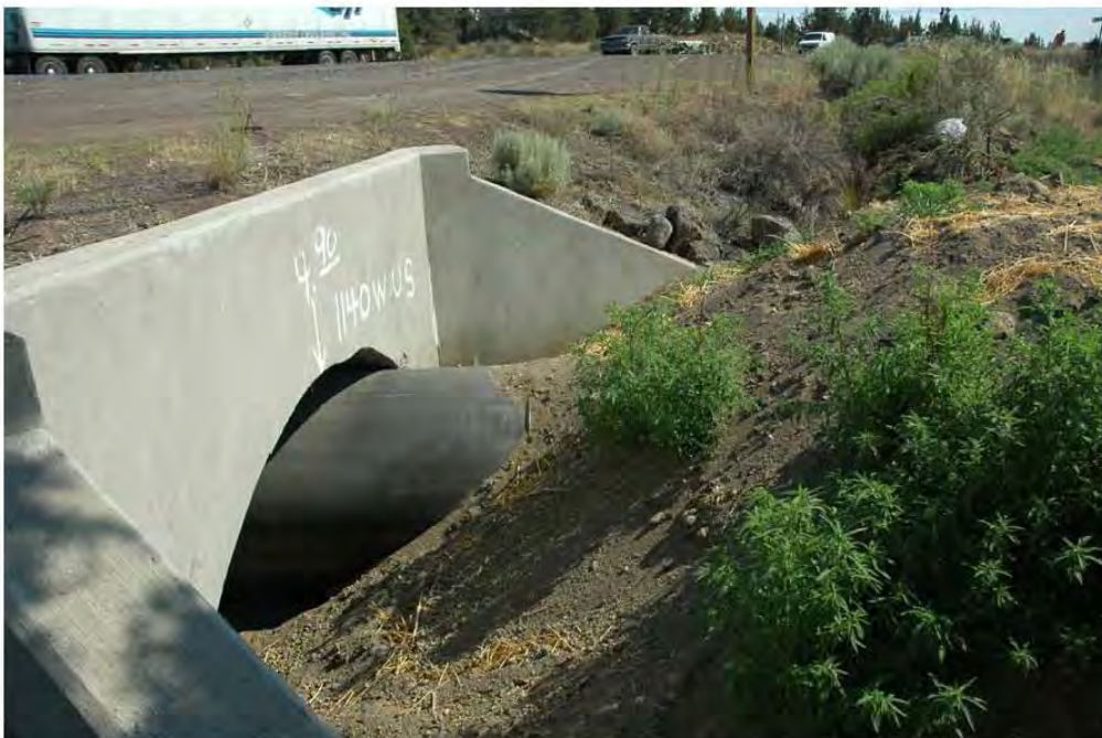
View: New culverts have been constructed at major roadways during recent piping activities. The view is towards the southeast.
