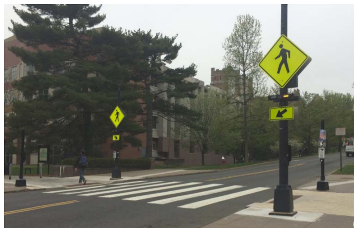
Figure 20: An Example of a Rectangular Rapid Flashing Beacon (RRFB)
