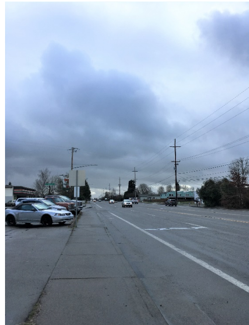
Highway segment near SE Lily Avenue with curb-tight sidewalk and no landscaping buffer
