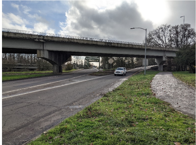
US 20/OR 34 Interchange and historic Marys River Bridge
