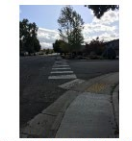
Looking south, SW Perkins Ave and SW 44th St intersection. Many students cross here and vehicles back up around the corner from the student pick-up line.
