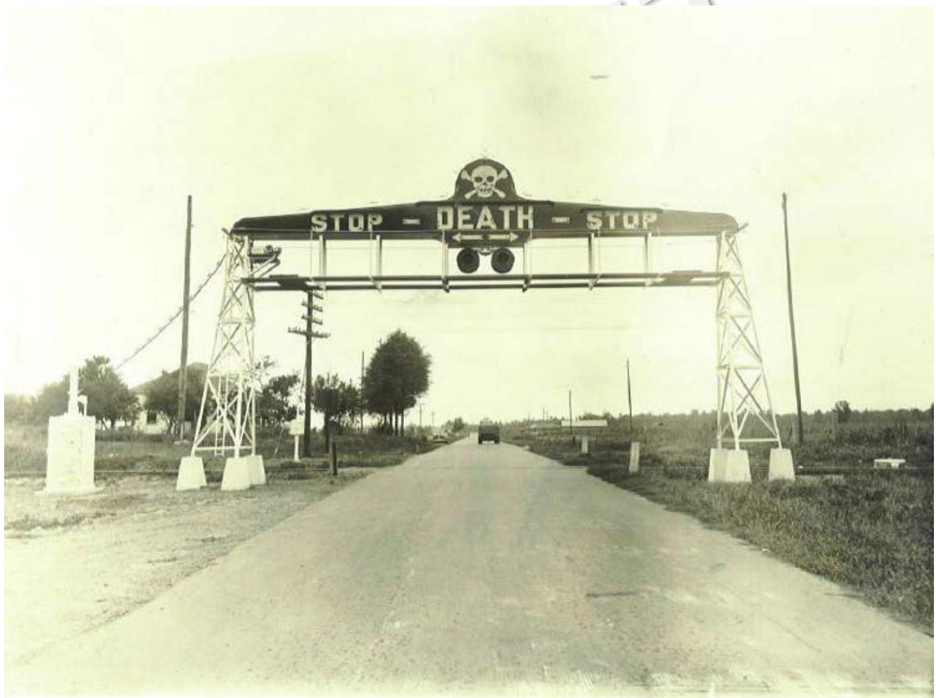
Early highway-rail grade active warning device.
