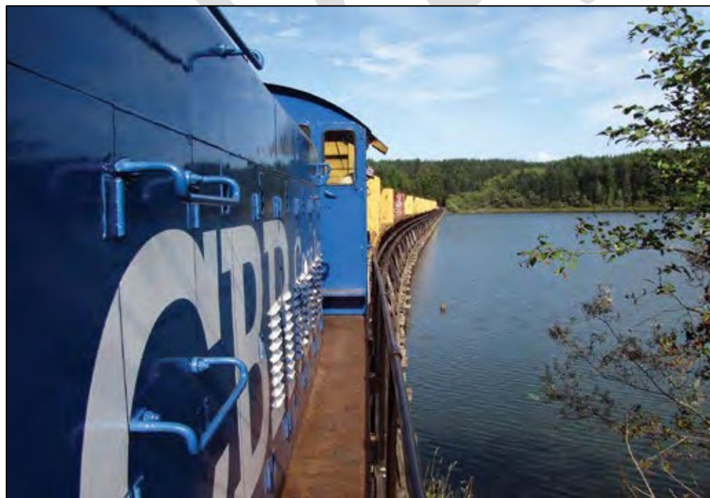
Figure 2-8. Coos Bay Rail Line train over the Siuslaw River Bridge
