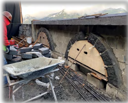
West portal wall concrete form
