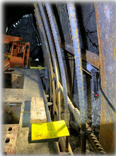
West portal wall concrete form
