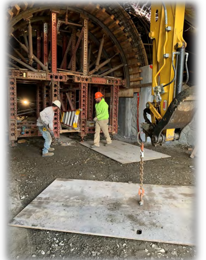
East portal structure frame form relocation
