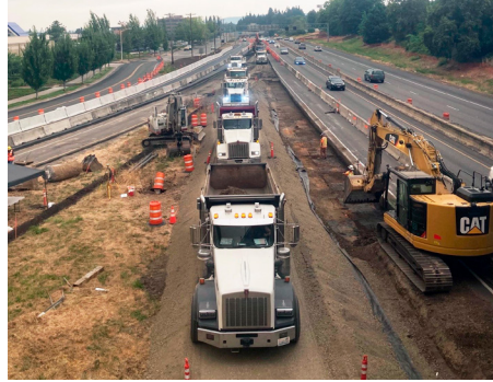
Dump trucks line up along OR 217 to haul away old pavement and top level of soil.
