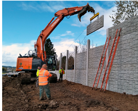
Crews place wall panels in the new sound walls along OR 217.
