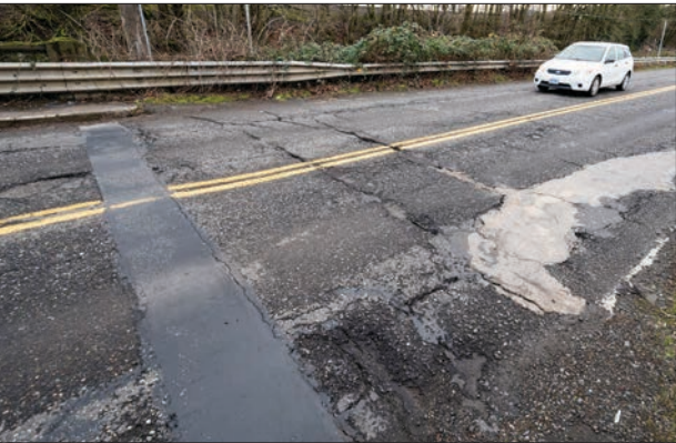
Current conditions of the bridge deck, which is deteriorating.
