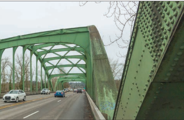
McLoughlin Bridge is in need of new paint to protect the steel structure and prevent corrosion.
