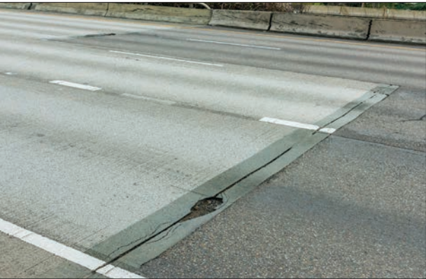
Rutting at the bridge joints.
