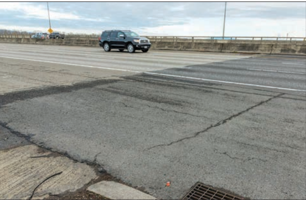
Poor pavement condition on the Glenn Jackson Bridge.
