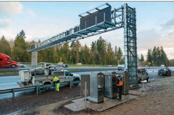
Workers perform maintenance on a VMS on I-205; these signs can display important traveler information.
