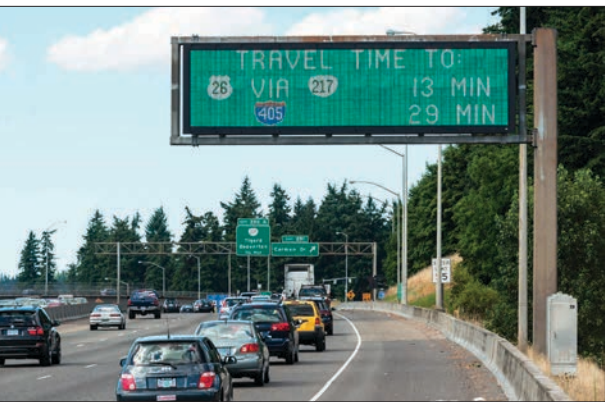
ITS infrastructure, such as RealTime data on I-5, enhances the operations of ODOT's system.
