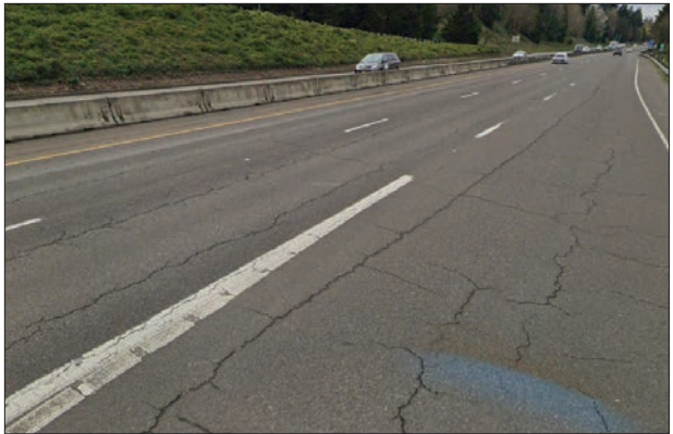
Cracking and rutting on the OR 224 pavement.
