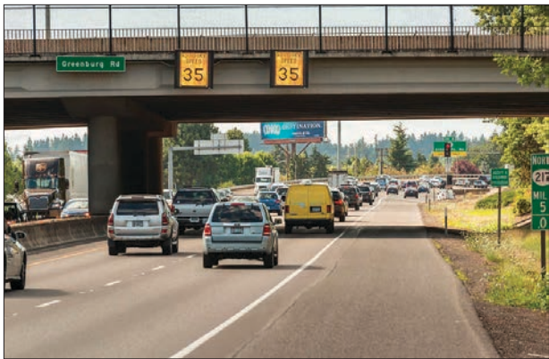
Example of Variable Advisory Speed Signs on OR 217.
