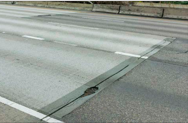
Rutting at the bridge joints.
