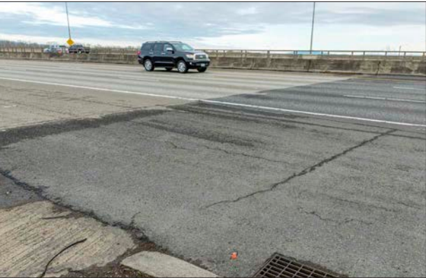
Poor pavement condition on the Glenn Jackson Bridge.
