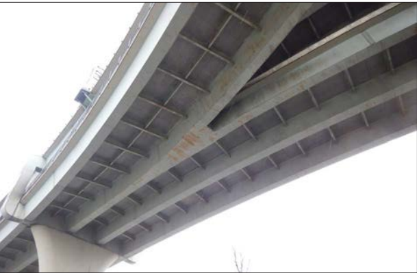
Rust on the underside of the Fremont Bridge ramps.
