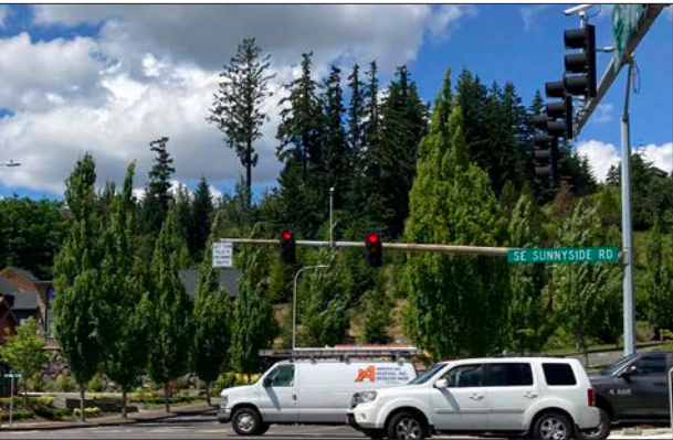
Traffic signals without reflective backplates on Sunnyside Road.
