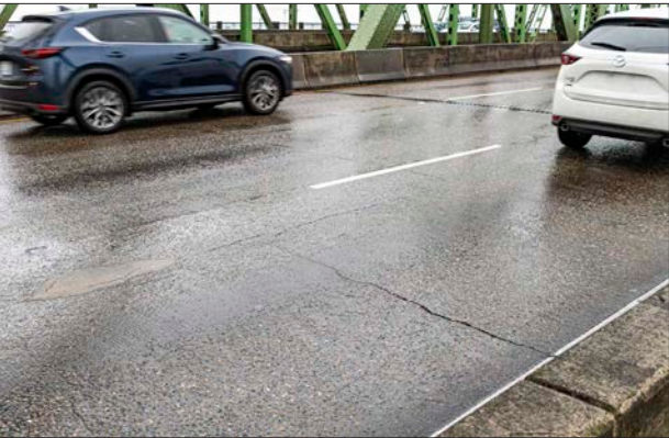
Cracked, worn bridge deck with exposed steel grid.
