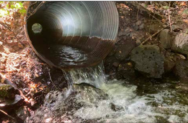
The existing culvert is too small for migratory fish to pass through.
