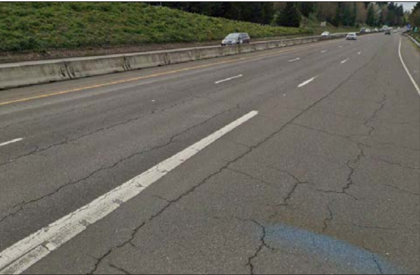
Cracking and rutting on the OR 224 pavement.
