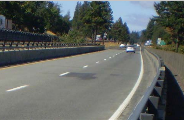
Large patches on the bridge deck surface from previous repairs.
