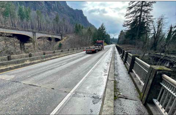
Rutting and wear on the Moffett Creek Bridge.
