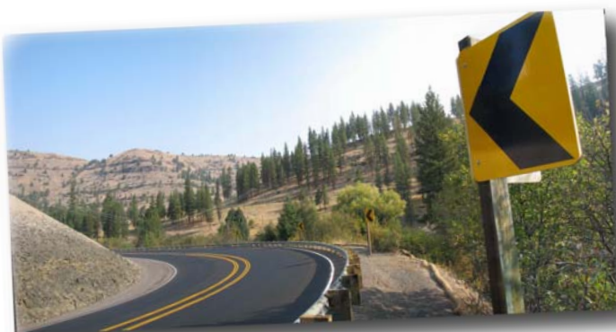
Newly widened curve at mile post 64.5
