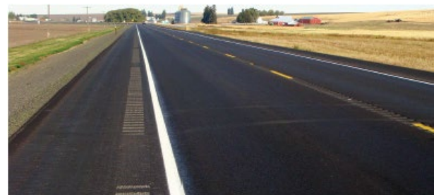
Figure 12. Graphic. Example of shoulder rumble strips (Source: FHWA).
