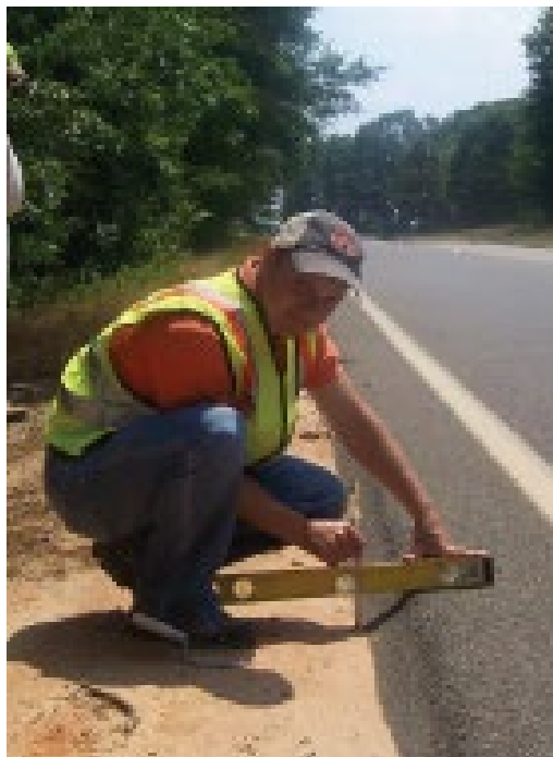
Figure 10. Graphic. Example of Safety Edge application (Source: FHWA).
