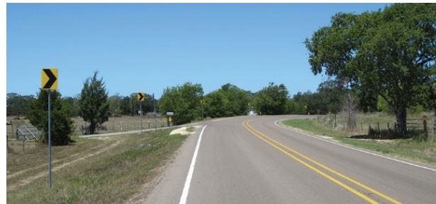
Figure 11. Graphic. Example of white edge lines, centerline raised pavement markers, and chevrons on a horizontal curve (Source: FHWA).
