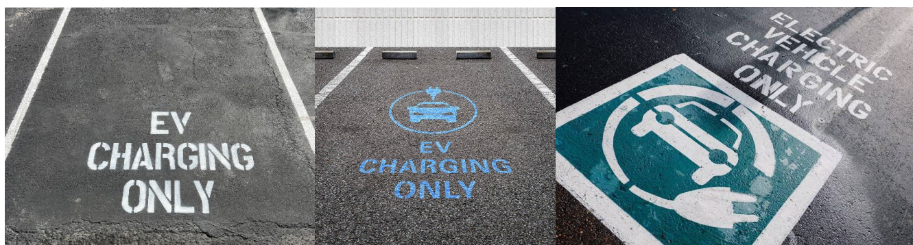
Figure 3 Examples of Acceptable “EV Charging Only” striping
