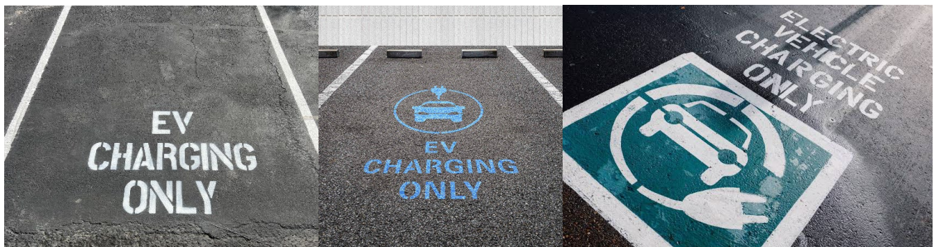
Figure 3 Examples of Acceptable "EV Charging Only" striping
