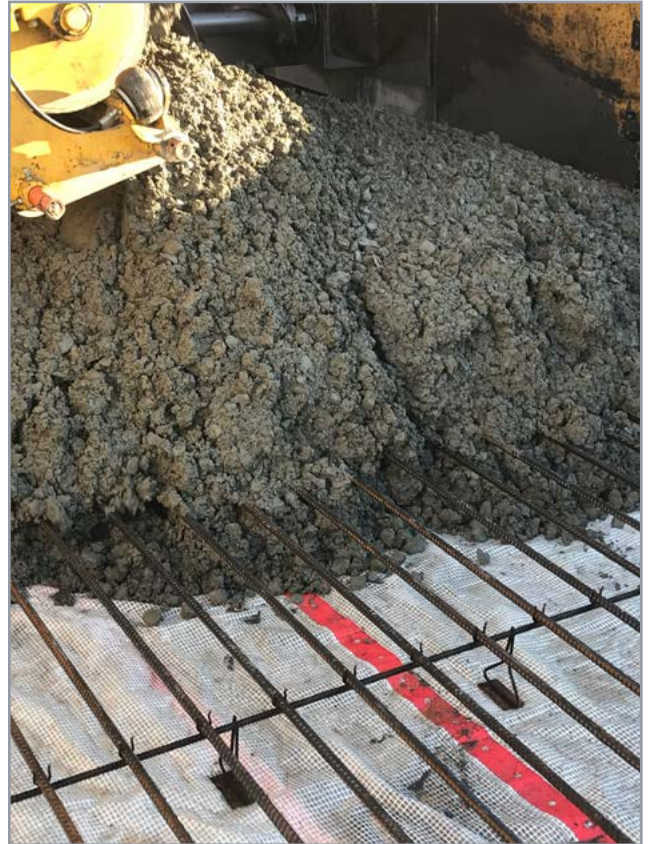
Fig. 6 – Low-carbon concrete installed in I-84 near Meacham.
