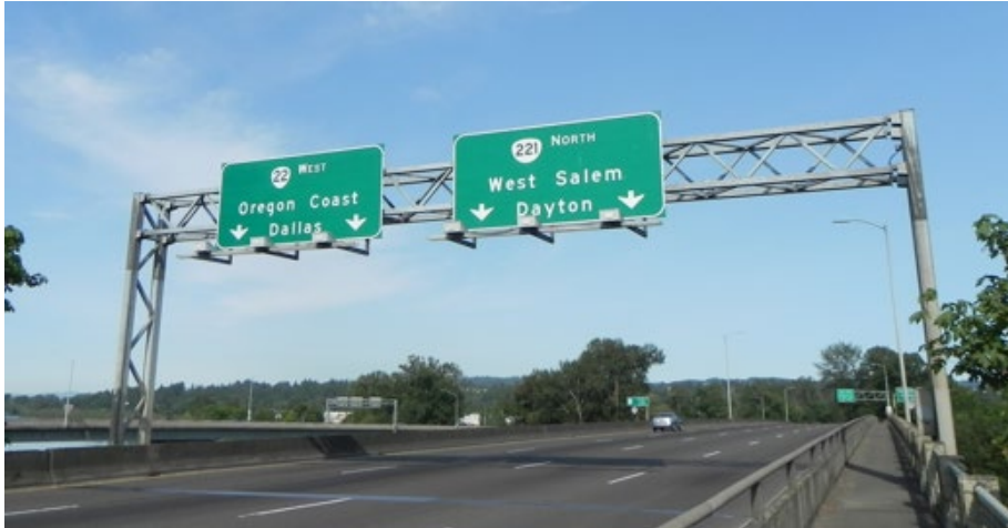
Figure 1: Truss Sign Bridge
