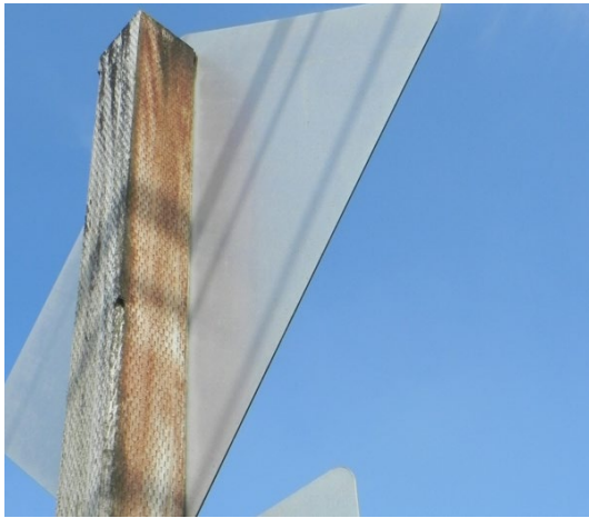
Figure 5: Wood Post for a warning sign
