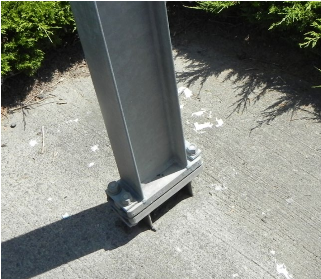
Figure 33: One support for a large sign that has multi-post breakaway supports
