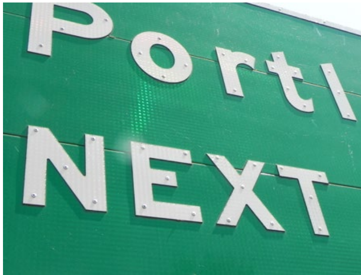
Figure 25: Demountable legend on extruded aluminum
