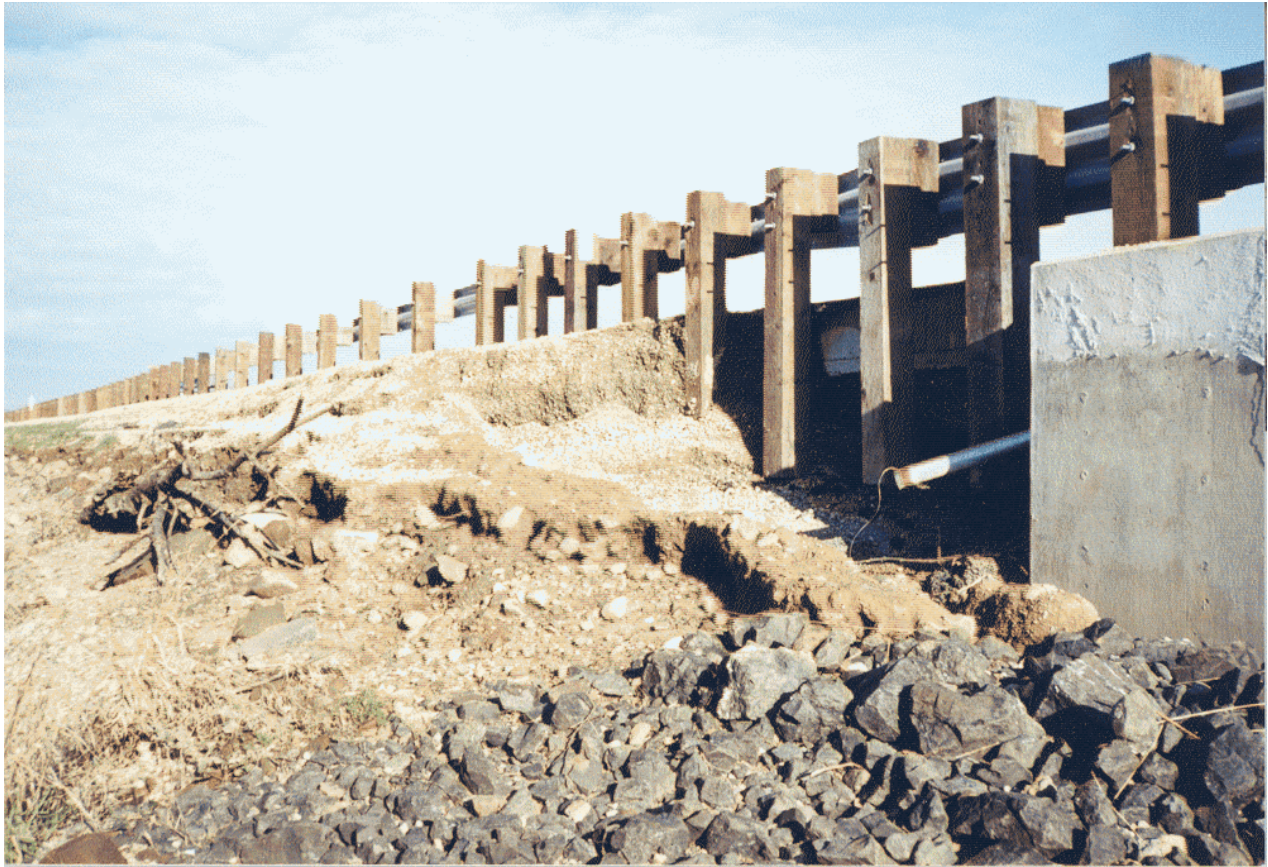
Figure 10-18 Undermined End Panel
