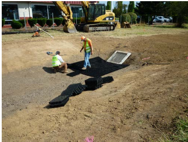
Swale with an access grid using porous pavers
