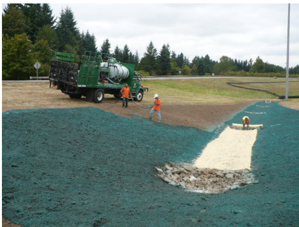
Figure 4 Biofiltration Swale (Southbound I-205 ramp onto Southbound I-5)
