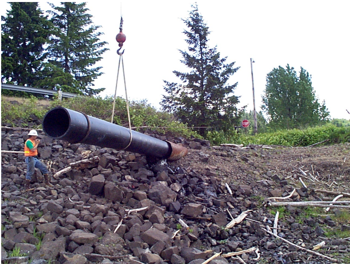
Figure 16-1 Sliplining with Fusion-Welded Continuous Pipe
