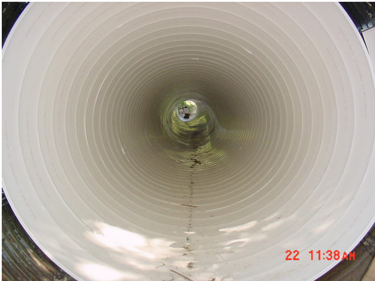
Figure 16-4 Spiral-wound pipe
