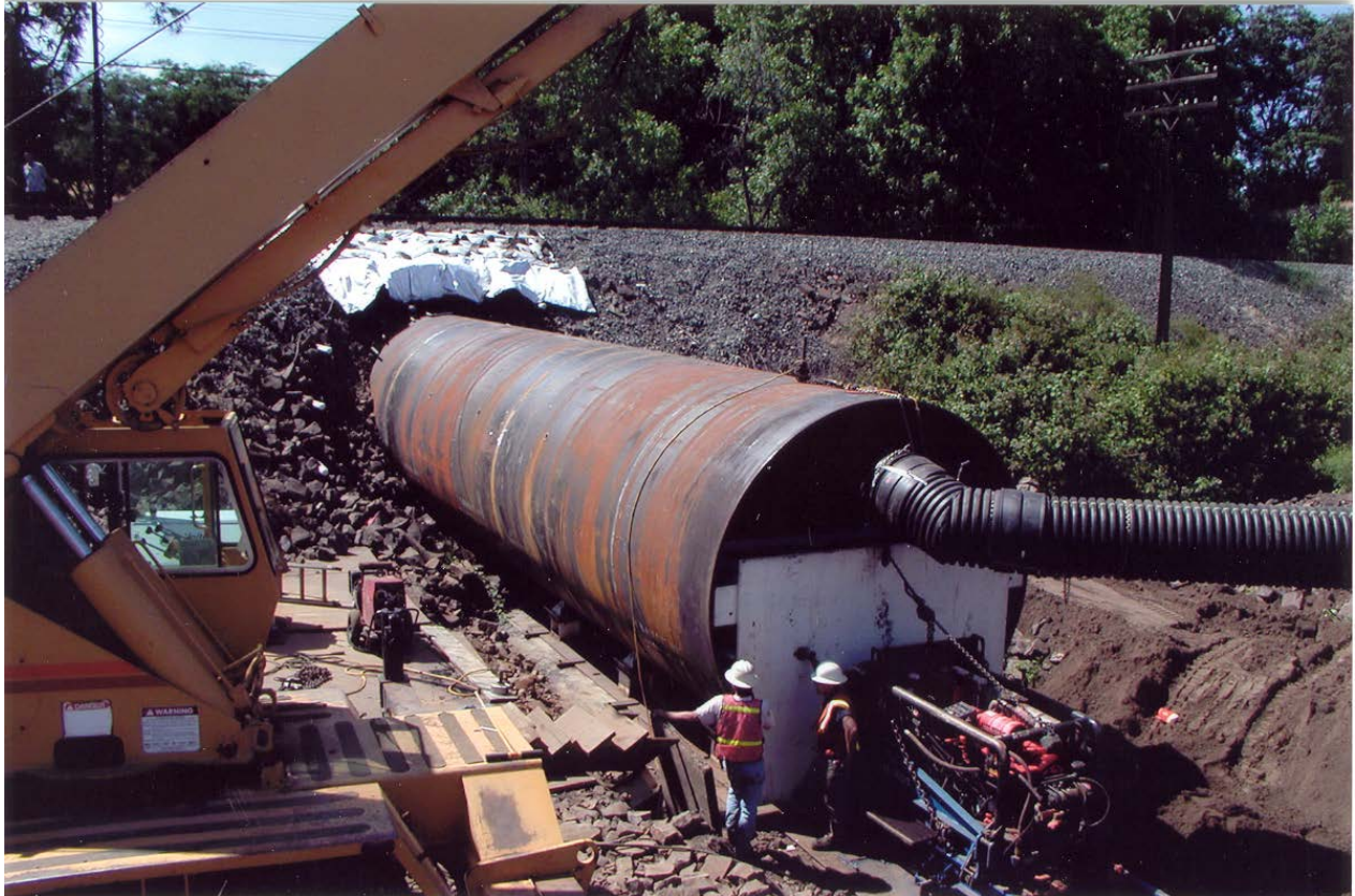
Figure 16-5 Pipe Jacking
