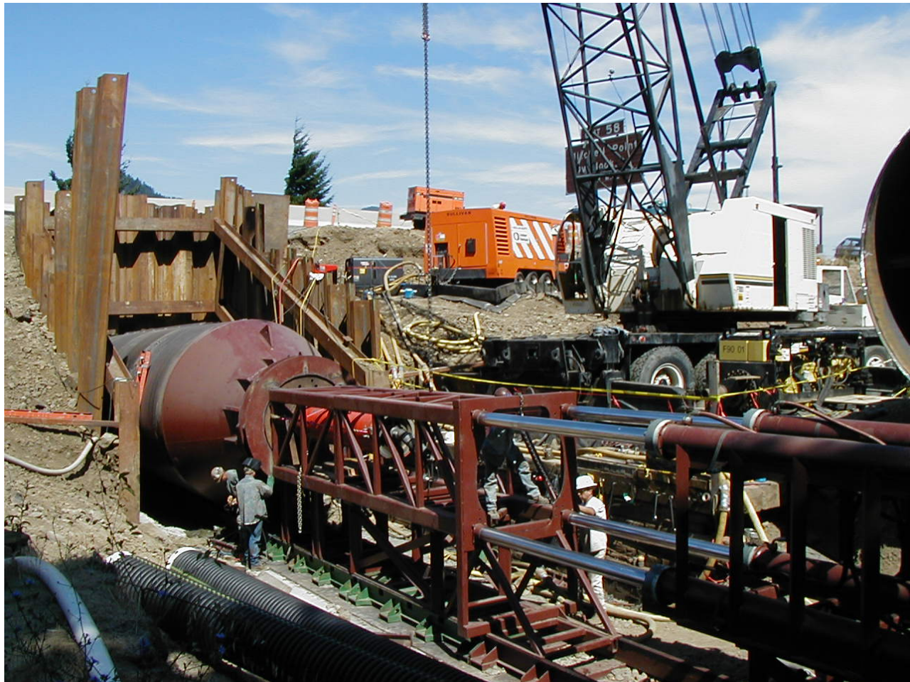
Figure 16-7 Pipe Ramming
