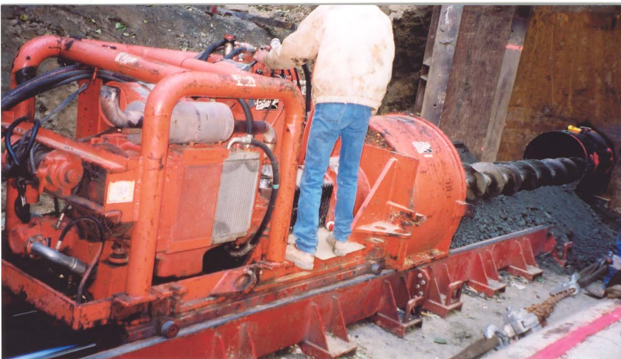
Figure 16-6 Auger Boring
