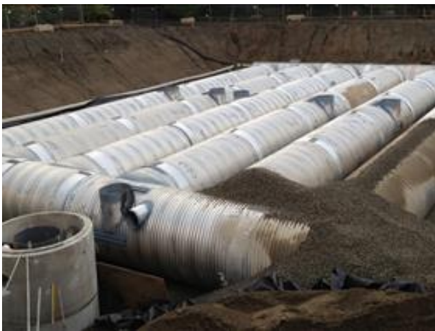
Figure 11: Contech CMP Detention and Infiltration System
