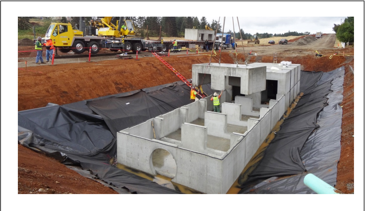
Figure 14: Installation of a detention vault
