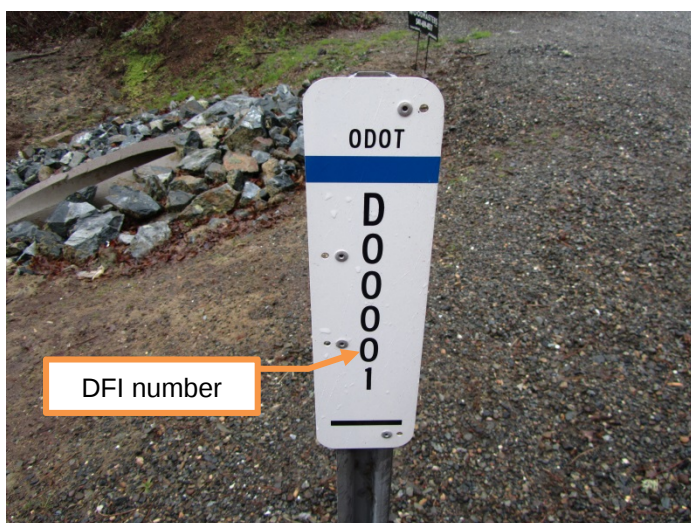
Figure 2: Type S2 marker detail
