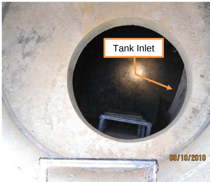
Figure 9: Top view of access manhole
