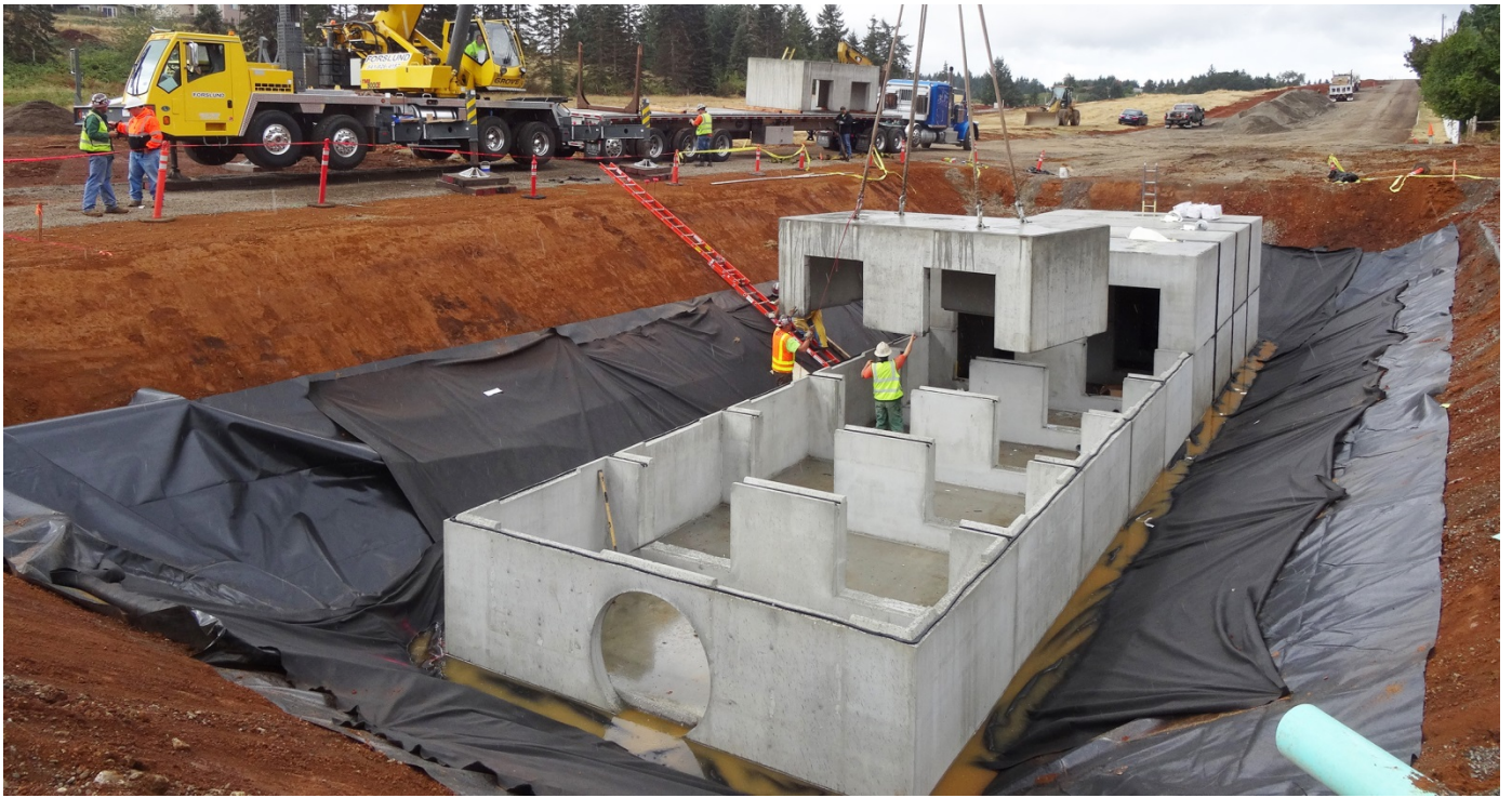
Figure 1: Installation of a detention vault
