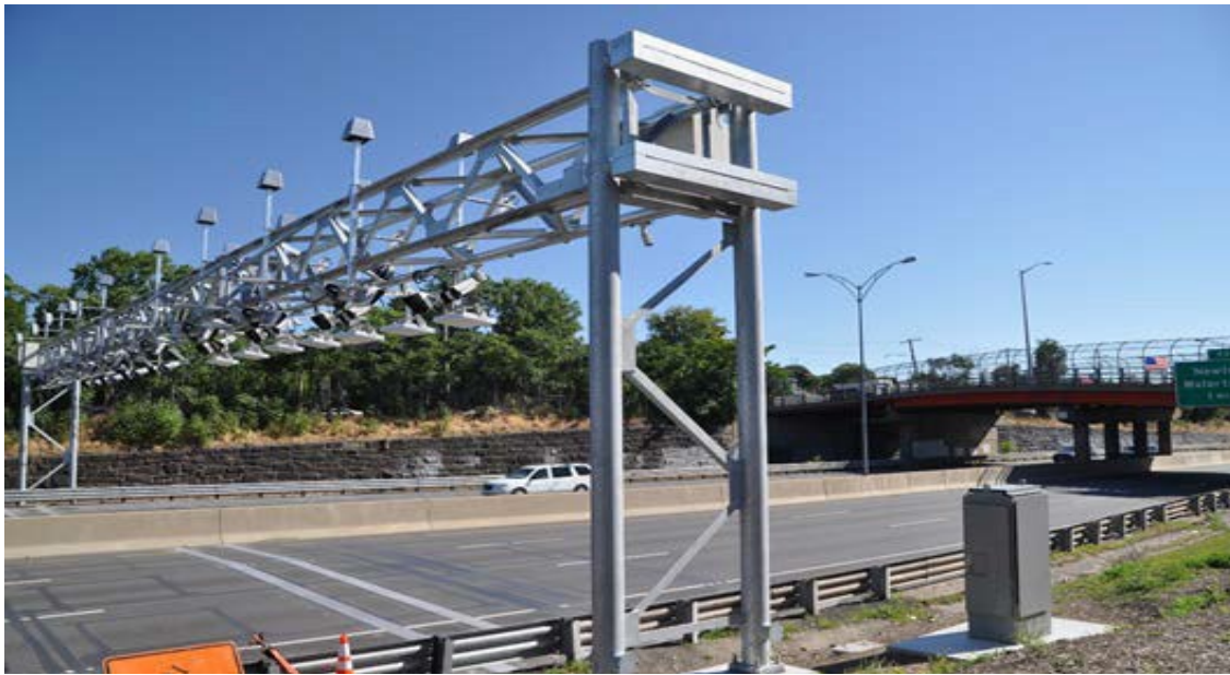
Figure 14 Massachusetts Turnpike All-Electronic Toll Zone and Gantry
