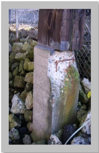
Figure 6.7 and 6.8: This under-designed oil terminal pier foundation (left) in area with high susceptibility for liquefaction and lateral spreading in the CEI Hub and the poor timber-to-concrete oil terminal pier connection and exposed rebar foundation (right) in the CEI Hub are considered inadequate (Source: DOGAMI photo)
