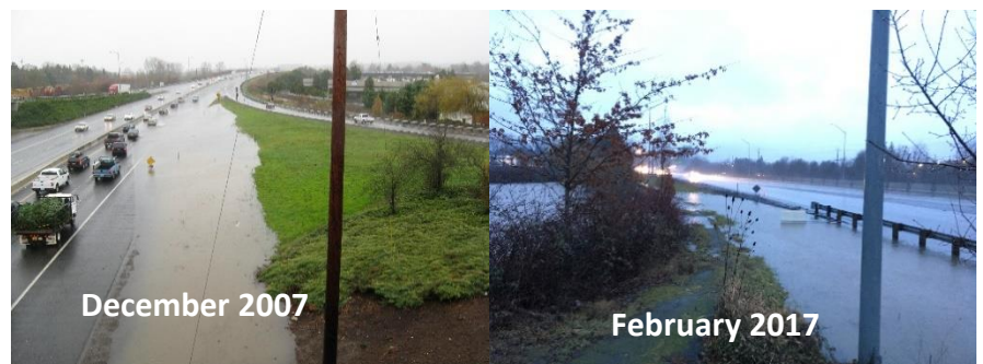
Figure C.2: Flooding on Hwy 217
