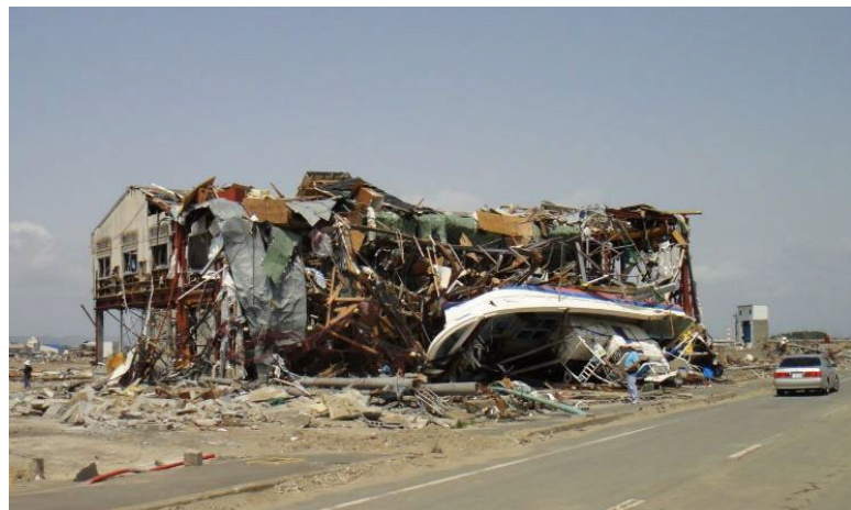
Figure 5. Natori, south of Sendai, Jaffe noted that damage indicated a 10-meter flow depth (depth of the water from the tsunami). (Public Domain, USGS)
