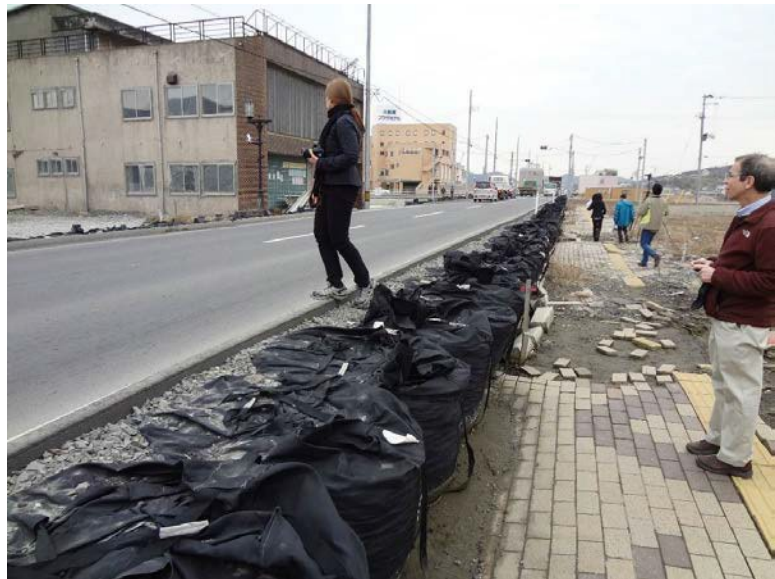
Figure 24. Compacted tsunami debris and sediment is used as a base to elevate roads in an area of Japan which experienced co-seismic subsidence. (Source: Rick Wilson)
