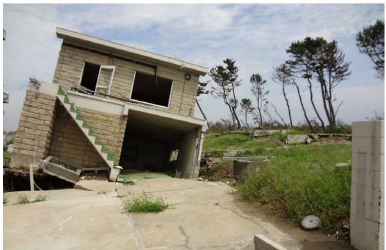
Figure 18. Sediment erosion around building foundation during the 2011 Great East Japan tsunami causes tilting of the structure along the Sendai plain in Japan. (Photo by Rick Wilson, CGS)
